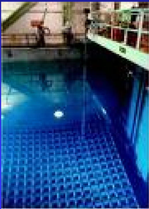
Spent fuel pond
